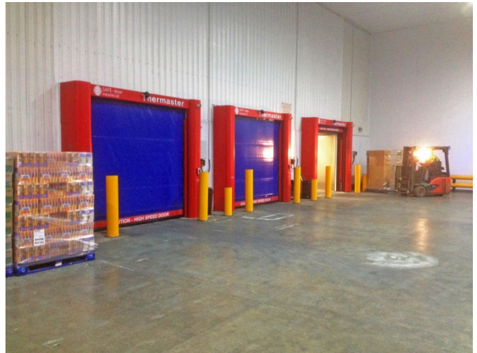
Image 2 – new Thermaster high speed doors
