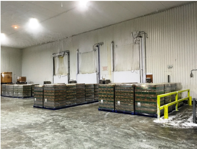
Image 1 – old solid panel sliding doors
